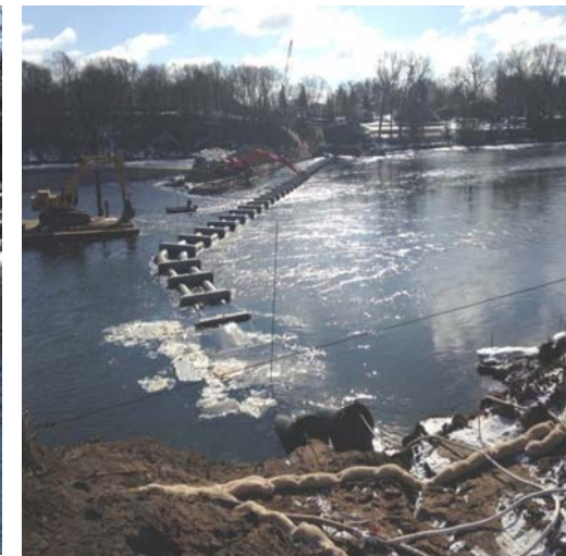
Mississippi River Force Main Project – Dual 42” FM HDPE fusion welded and floated across the river. Anchors set and pipe slowly sunk from west to east.
