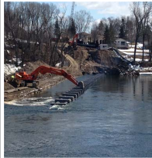
Mississippi River Force Main Project – Dual 42” FM HDPE fusion welded and floated across the river. Anchors set and pipe slowly sunk from west to east.
