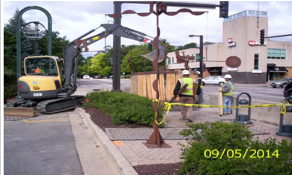
Edina - Ring Beam and Lagging - Top 4' Being Placed on Grade
