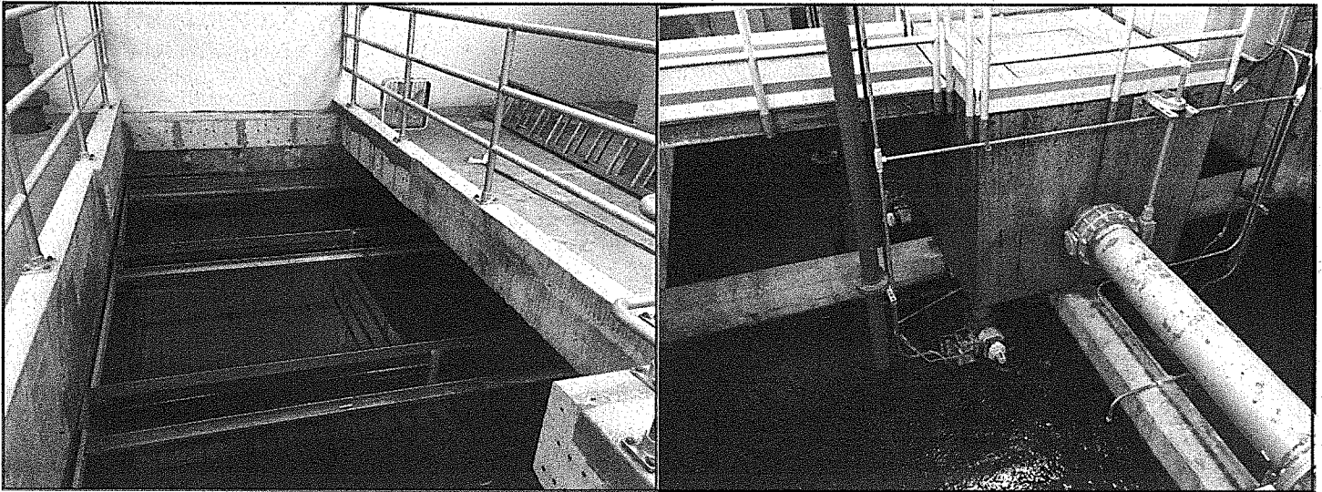
Plate settlers (left) were added to the treatment process in Ortonville to reduce the load on the filters (right).
