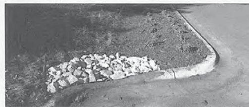
One of six bioswales installed along 3rd street.
