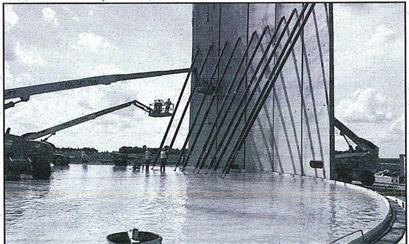
Wall panels are installed for the Rock County reservoir.
