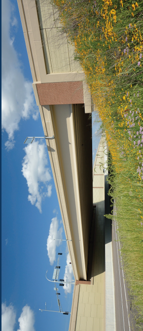
Armstrong Boulevard Bridge (Bridge 02007), City of Ramsey
