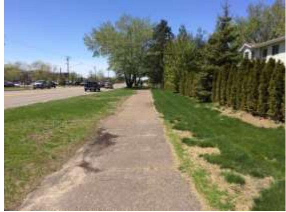
Just west of Quincey ST. NE – edge failure (looking west).
