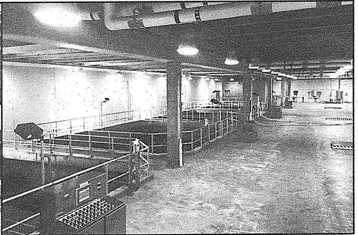
The softening basins (left) and filters (right) at the Vermillion plant. The pipes on the filters have been stubbed to allow for expansion with an addition to the building to the north.
