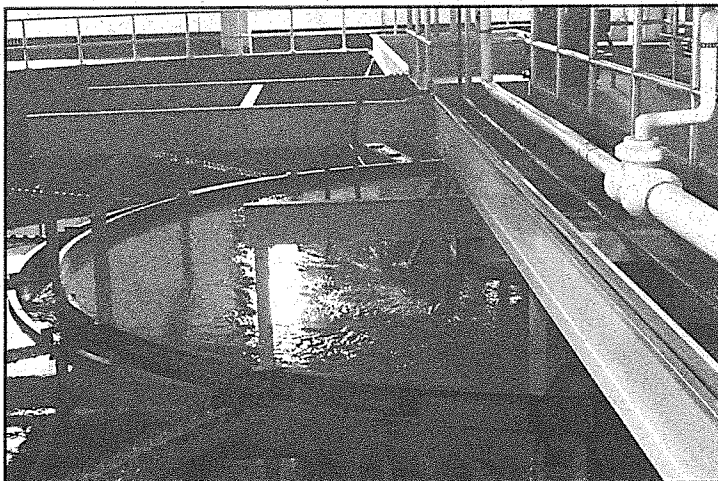
The softening basins (left) and filters (right) at the Vermillion plant. The pipes on the filters have been stubbed to allow for expansion with an addition to the building to the north.
