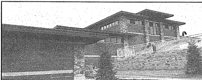
The backwash holding tank is partially surrounded by the rock wall on the right.
